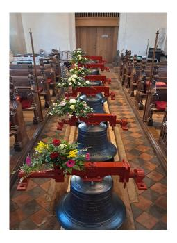
On Tuesday 11<sup>th</sup> March, the six new bells were lifted from the church floor and safely installed in the bell frame at the top of the tower, their new home for many decades to come. All the fittings were then added over the next couple of days: clappers, wheels, pulleys, runners, sliders, stays and ropes.
